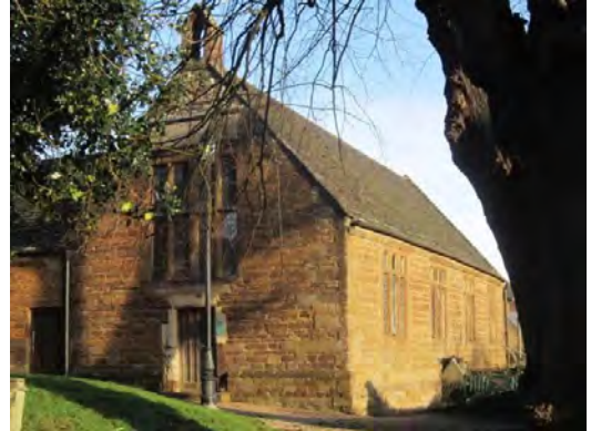
The Old School Room
