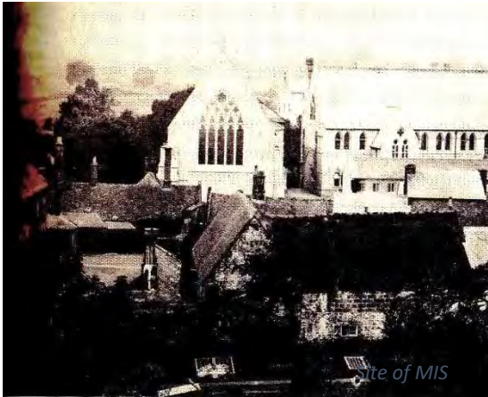
Building Site for MIS
